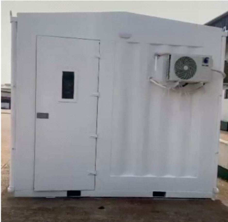
Mobile substation for MCC Panel (Drive, LV Panel and Transformer)
